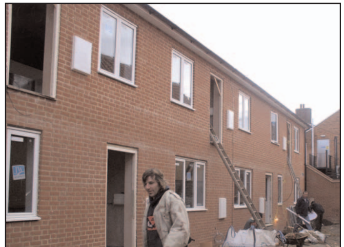
The exterior of the residents flats
