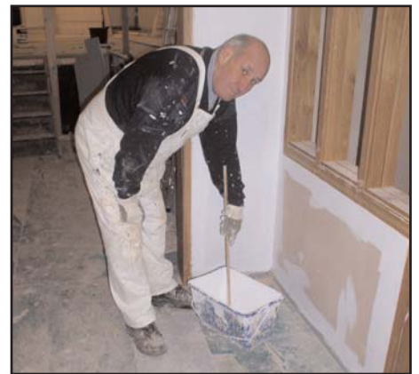
A Malthouse painter mixing limewash, ready to add the Ladylane Yellow colour to it.
