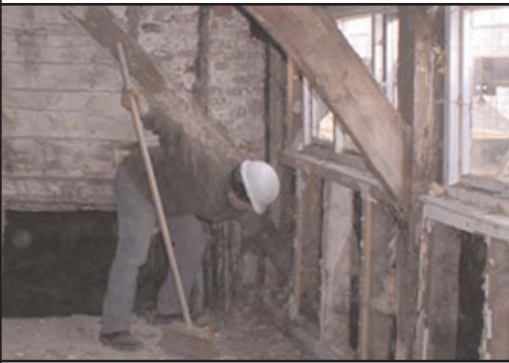
A worker clears the site
