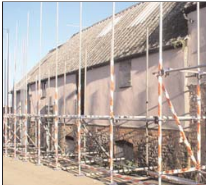
The Malthouse with protective scaffolding
