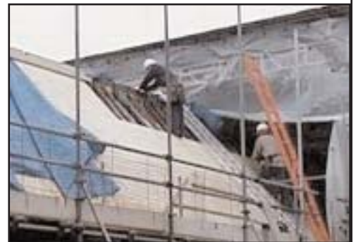
A worker gives the roof its protective cover
